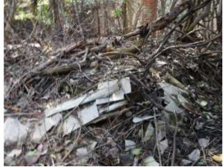
**Photo 30:** View of transite siding and debris associated with the dilapidated residence in the southeastern portion of the Site.
