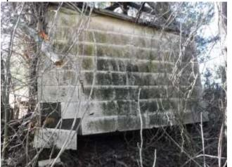
**Photo 27:** View of dilapidated outbuilding in the southeastern portion of the Site. Note the suspect asbestos containing transite paneling.
